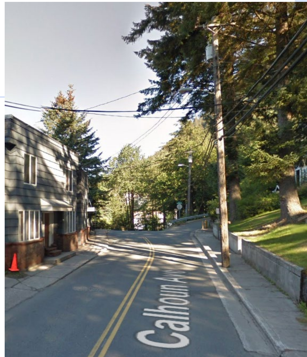
Typical overhead transformer and service drops – across from 925 Calhoun
