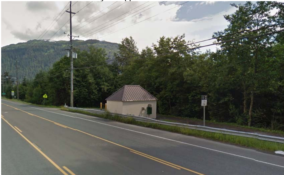
Gruening Park Pump Station Generator Building
