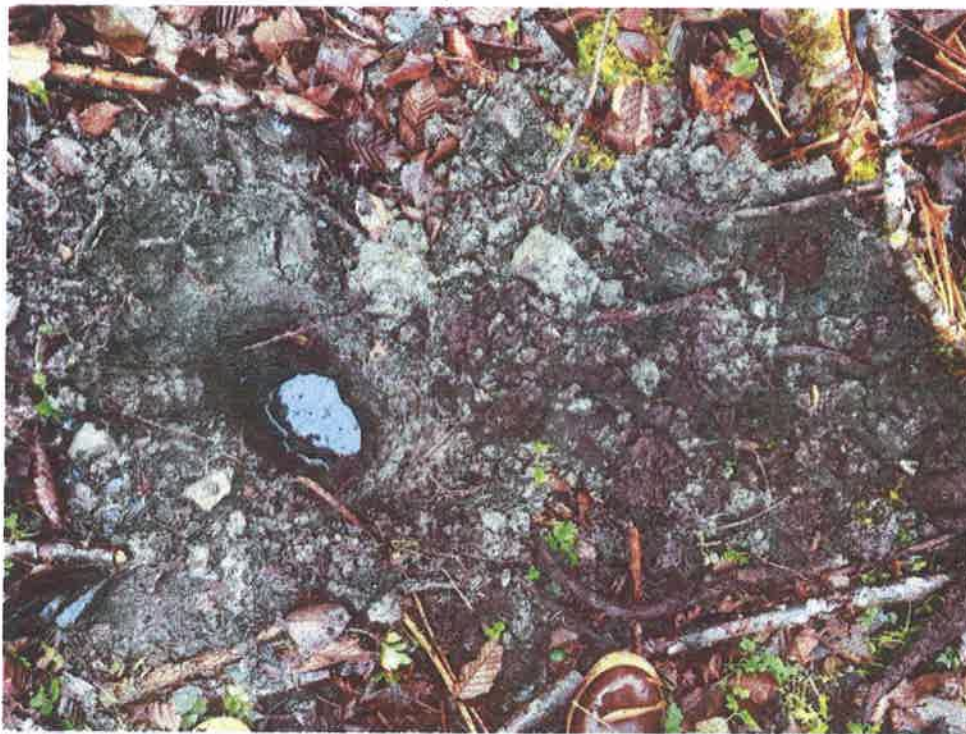
Photo 5 - Eroded fill material with silts and gravels over native organic soils at the toe of the fill pad.
