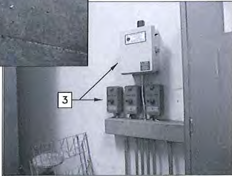
5B EXISTING AERATOR AND UV SYSTEM CONTROL PANELS NOT TO SCALE - USE DIMENSIONS IMG_7124
