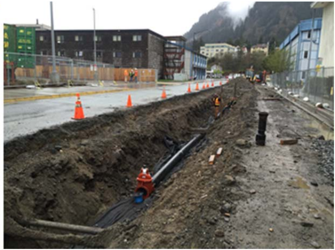
HDPE waterline installation on Whittier Street
