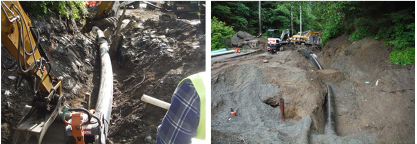
HDPE waterline installation at Cope Park
