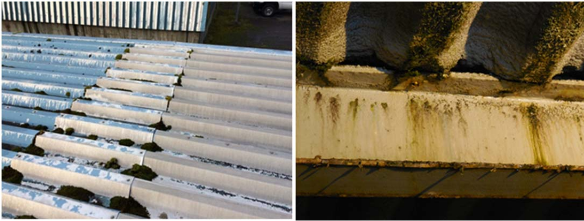
Left to right: exposed exterior fasteners on JDTP digester building roof; interior corrosion to clarifier building roof
