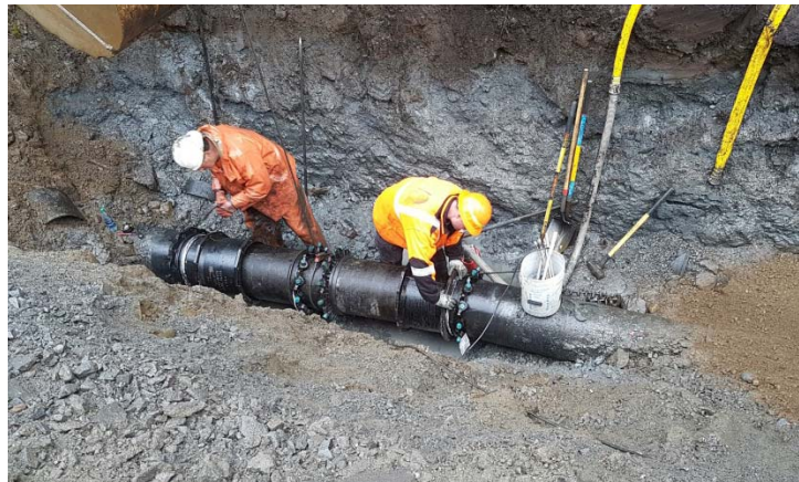
Water main line break and repair near Pt. Lena Loop Road
