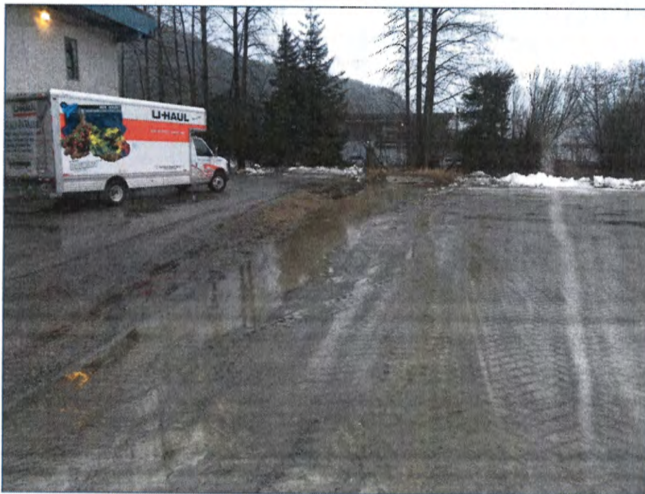
Figure 2. The Edward K Thomas Building project site during a rain event with stormwater run-off draining towards Jordan Creek, which is in the background.
